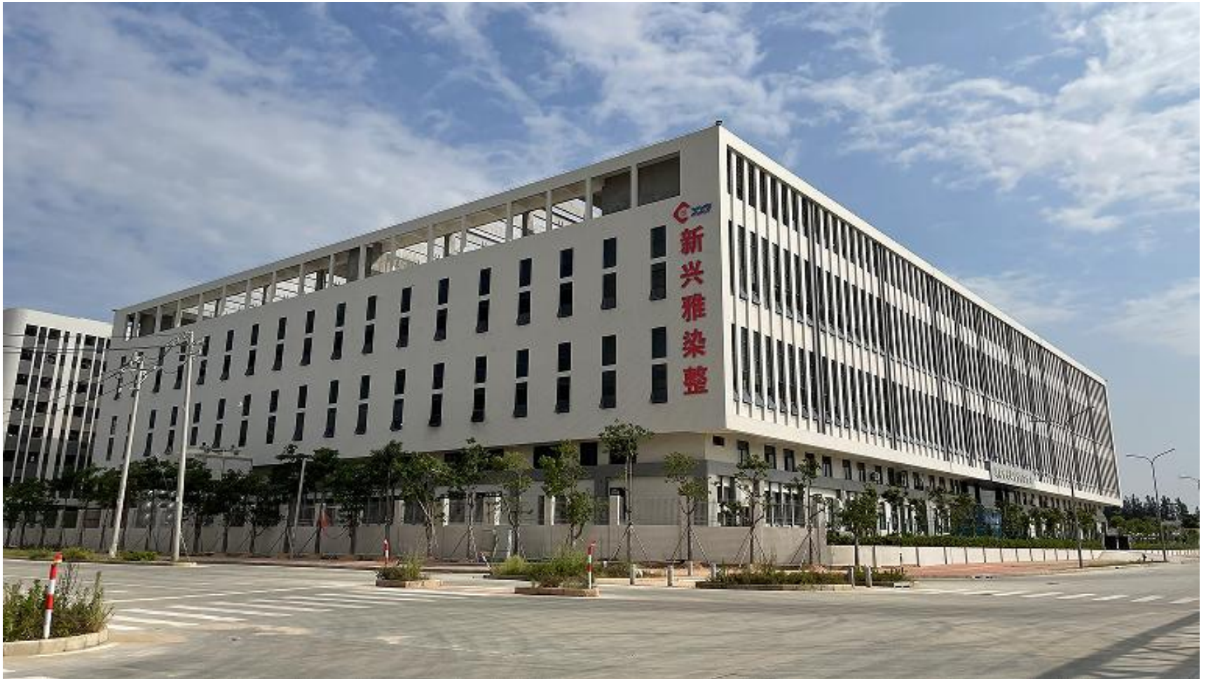
Side View of Dyeing & Finishing Mill
